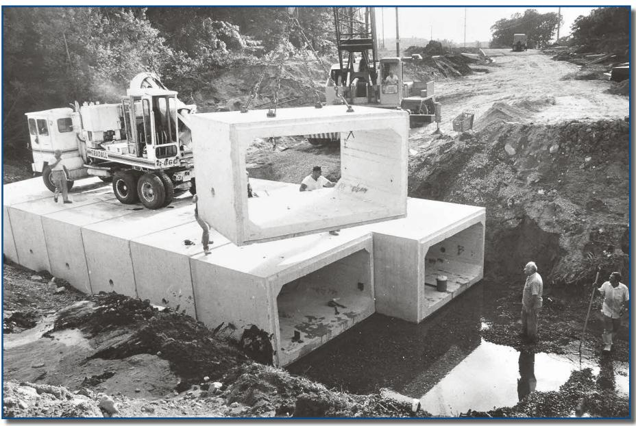
Installing culvert on Flutie Pass, Natick MA, September 3, 1985
