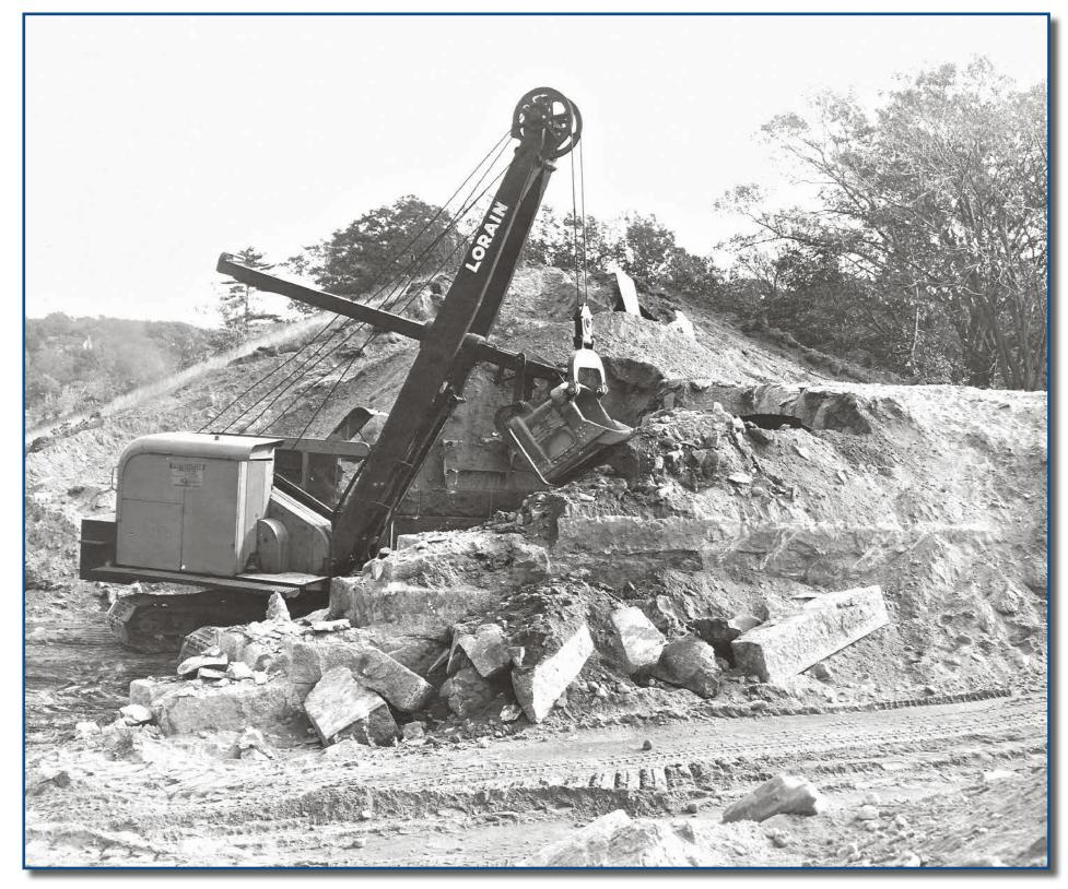
Northeastern Construction Company, Lorain shovel removing aqueduct bridge, Cedar St., Wellesley, MA, 1950s
